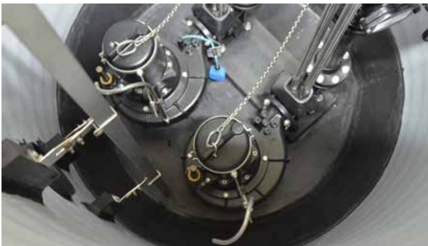
► Pumps with flushing tube
